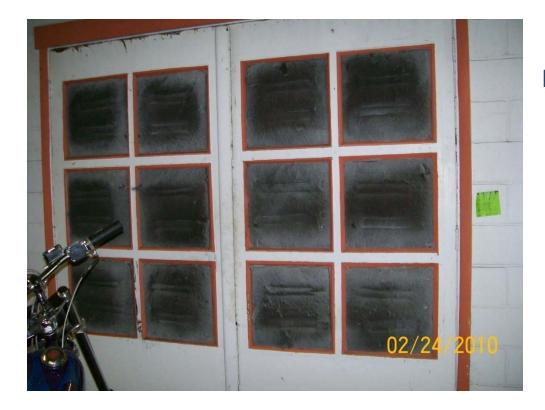
Paint booth filters can become hazardous waste if the paints being used contain heavy metals.
